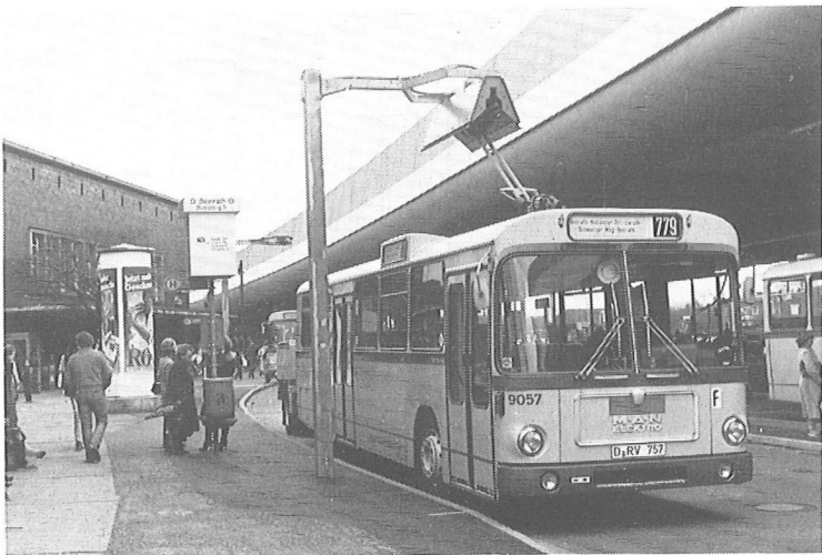
Fig. 6: MAN-Battery-Powered Urban Bus supplied by "Short Term Intermediate Recharging"
