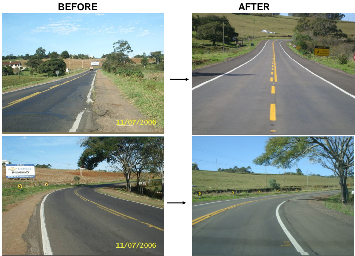
Figure 10. Image Before and After the Engineering Measures at 55 km of RS 030 km
