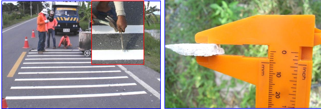
Figure 2 Installation of TRSs
