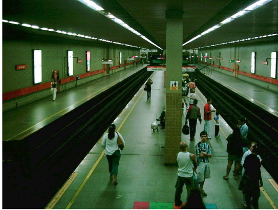
Figure 7: Botafogo Station – View 1
