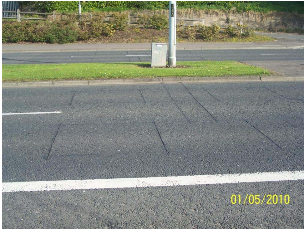
Figure 2 – Main data collection sites (inductive loops and the processing unit located in the median)
