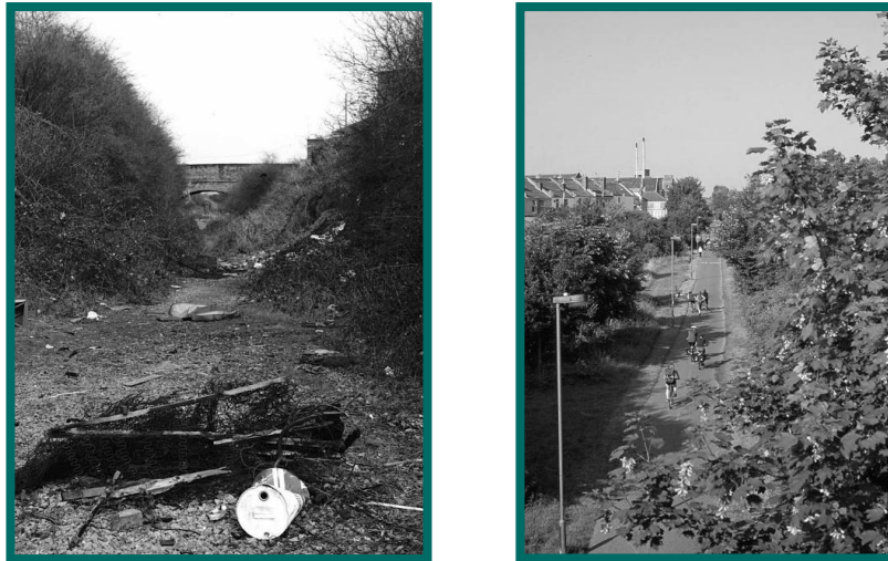
Figure 1: The Bristol and Bath Railway Path prior to development into NCN Route 4 now carrying some 1.7 million journeys a year (photos courtesy of Sustrans).
