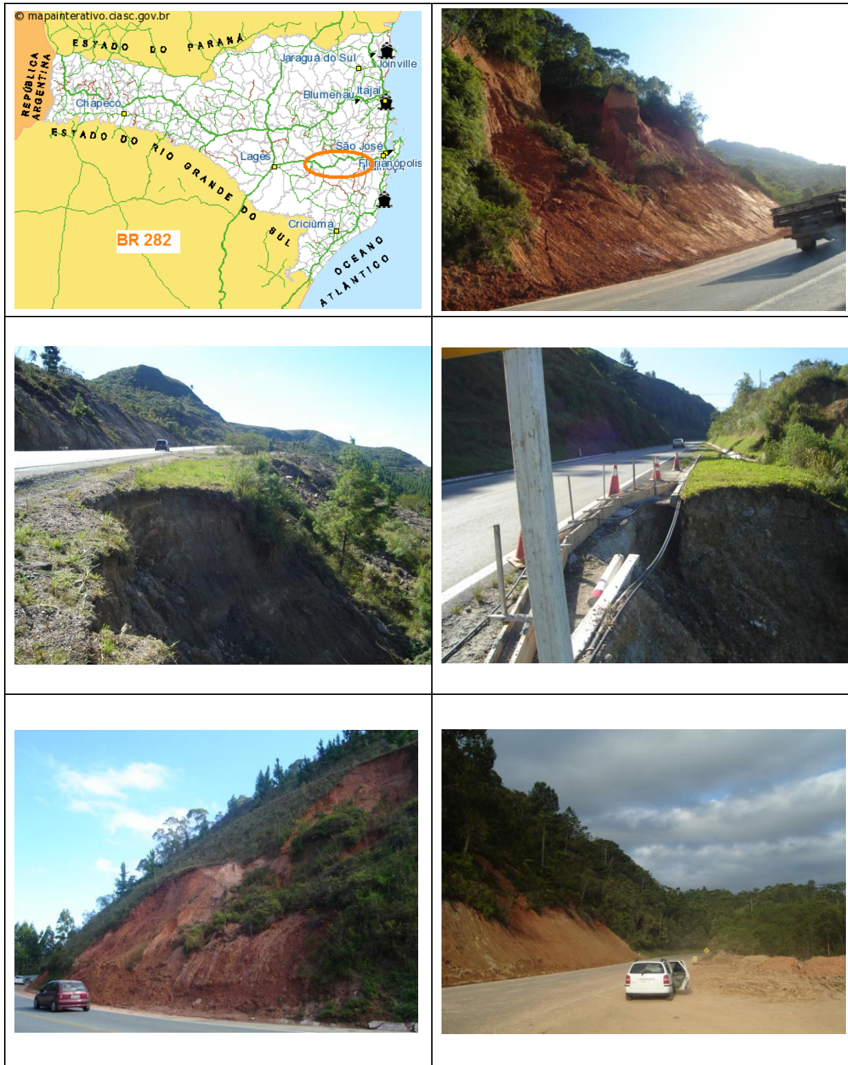
Picture 7 – Pictures of mass movement phenomena in different spots of BR 282, occurred during the rain of November, 2008. Date: December/2008.
