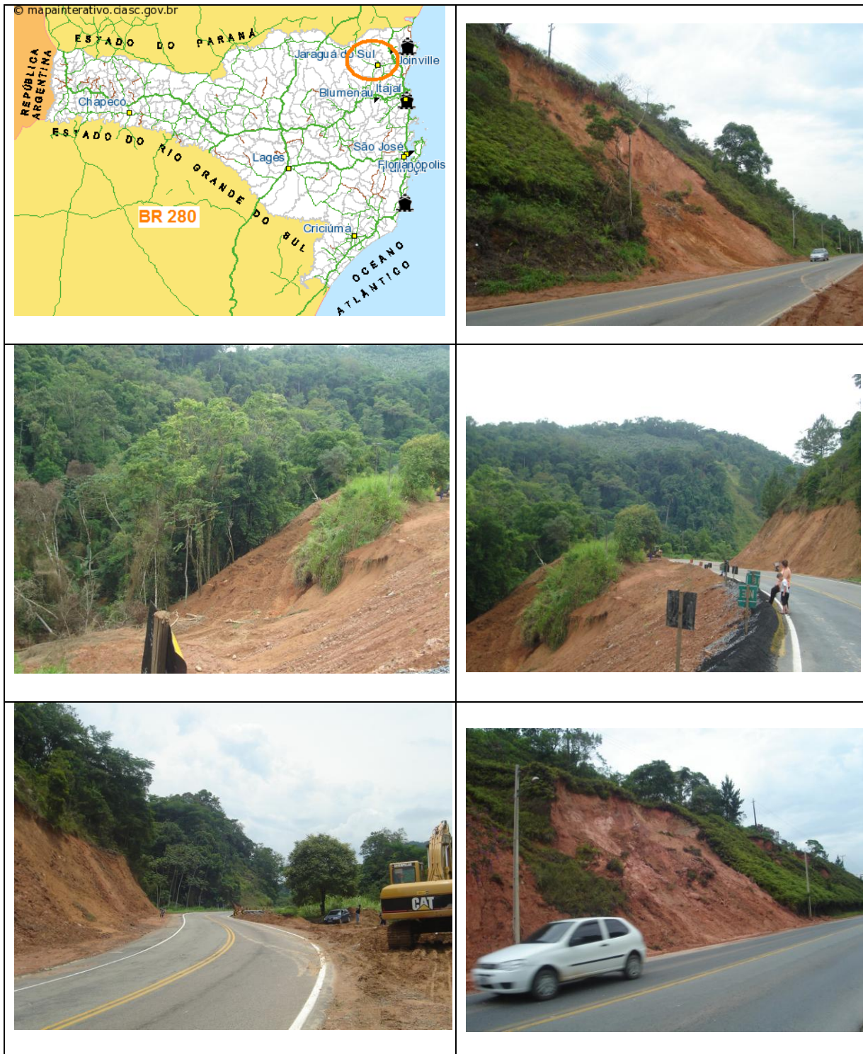
Picture 9 – Pictures of mass movement phenomena in different spots of BR 280 occurred during the rains in 2008. Date: Dec/2008
