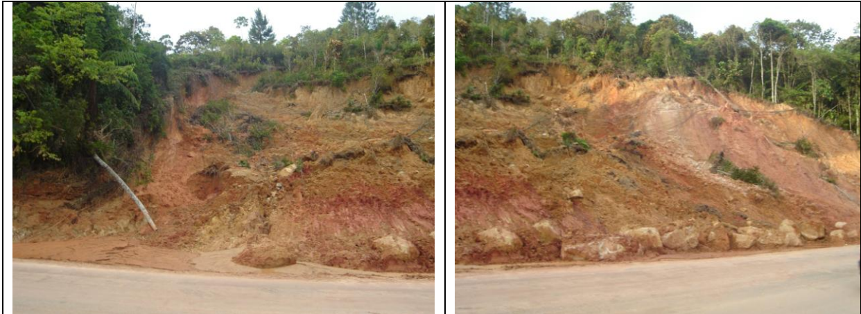
Picture 8 –Pictures of mass movement phenomena in BR 282 (area of Great Florianópolis), occurred during the rains of 2008. Date: dec/2008.
