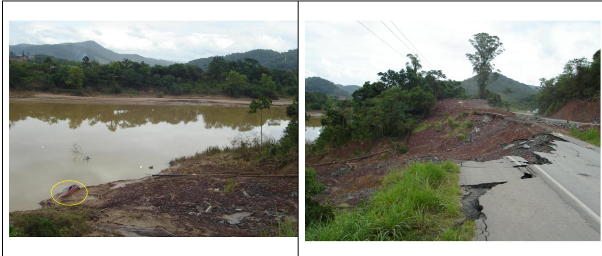
Picture 6 – Pictures of mass movement phenomena in BR-470, on the banks of Itajaí-Açu river after the rains of Nov/2008. Note the car in the river. Date: December/2008.
