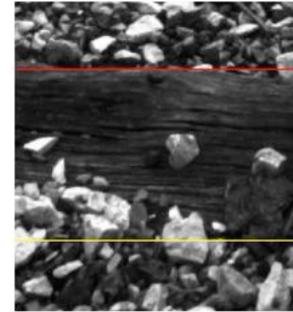
B: Tie Location Found Using Tie Template
