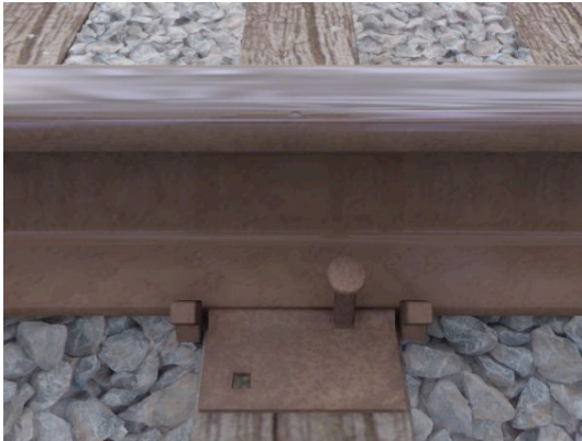
A: Lateral view showing view of simulated track and tie plate
