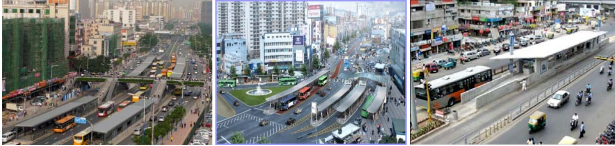
Figure 16. Contrasting approaches to pedestrian access to median-station BRT: Guangzhou (left), Seoul (middle), Ahmedabad (right). Sources: ITDP China, Cervero and Kang (2012), and author's photo.
