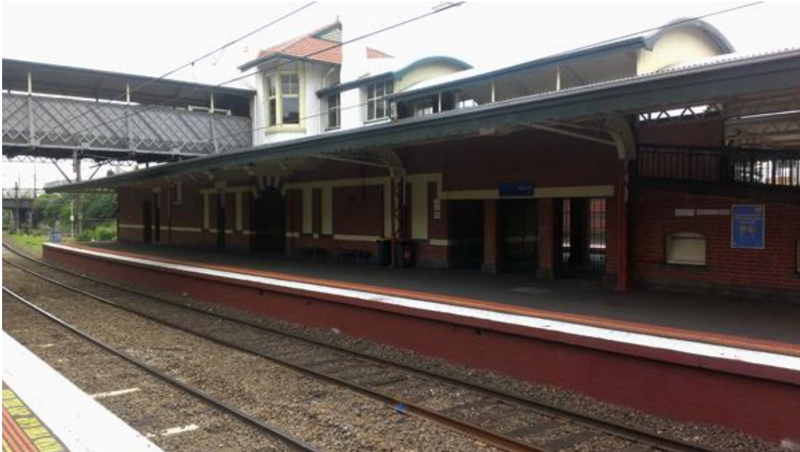
Fig. 4 Heritage listed Malvern Station, Melbourne (Moug 2012)
