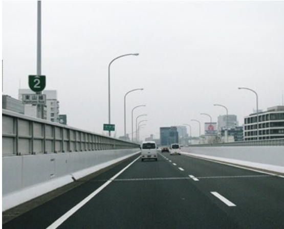
Figure 2 – Standard cross section of NEX Layout: 1.5m(shoulder)+3.25m(lane)×2+0.5m(curbside)
