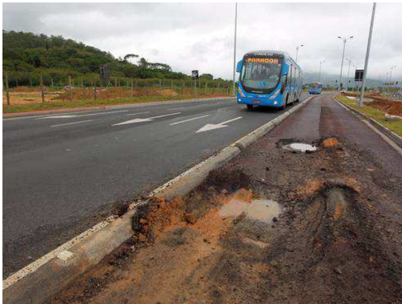
Figure – 3: Picture of transoeste BRT lane degradations'. Sources: Journal O Globo (06/01/2013). Available on: http://oglobo.globo.com/rio/inaugurado-ha-6-meses-corredor-transoeste-sofre-com-buracos-7207730#ixzz2Hl0fDWcv (Consulted on 13 March 2013)
