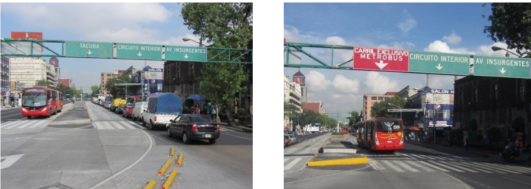
Figure 14. Overhead signs before and after interventions at Puente de Alvarado Street.
