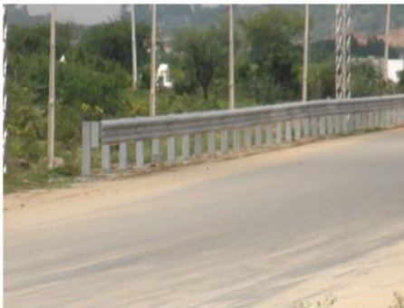
Fig. 10: Crash Barrier end treatment was not proper and High edge drops are potential for accidents.
