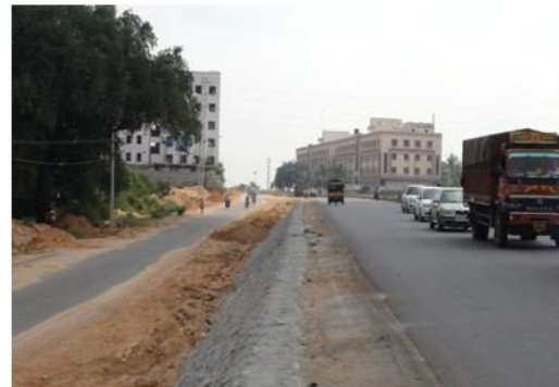
Fig. 10: Crash Barrier end treatment was not proper and High edge drops are potential for accidents.
