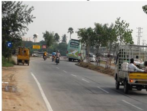
Fig 3. Diversion (RHS) from Hyderabad to Yadagiri use blinker for enhancing the safety at night and adopt diversion as per IRC specifications
