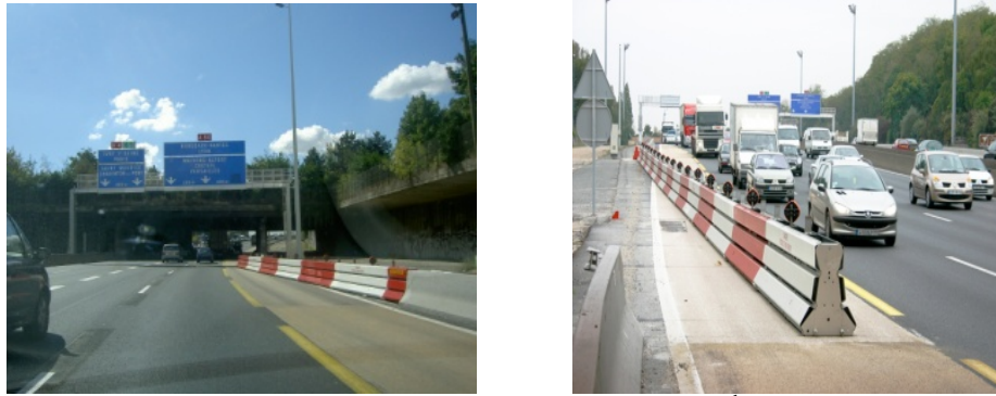
Fig. 2. The weaving A4-A86 section, eastbound with the 5 th lane, open and closed
