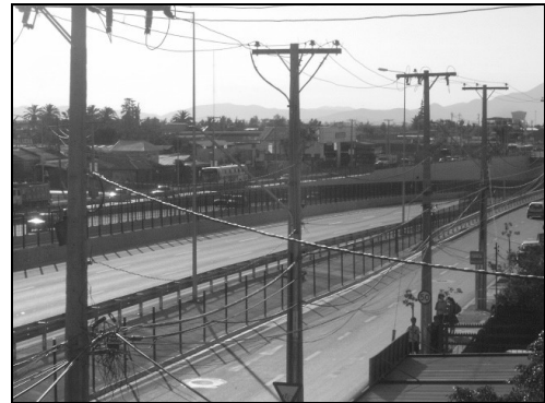
(b) Barriers to prevent pedestrian crossings
